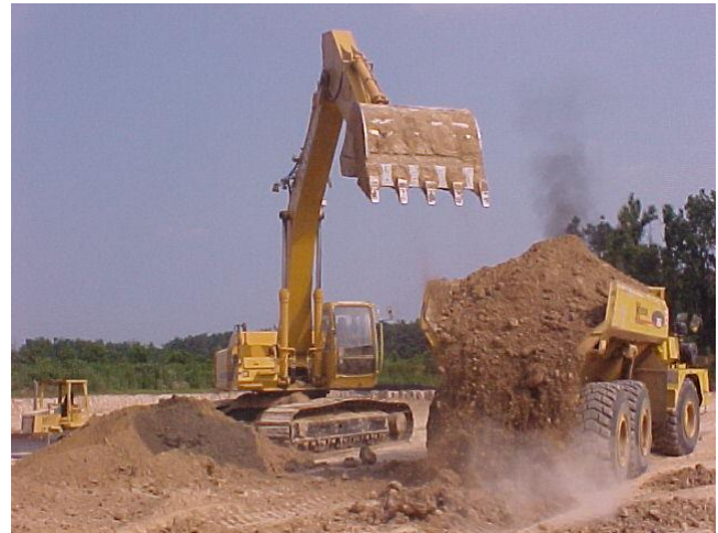
Borrow soil is loaded for impoundment closure
